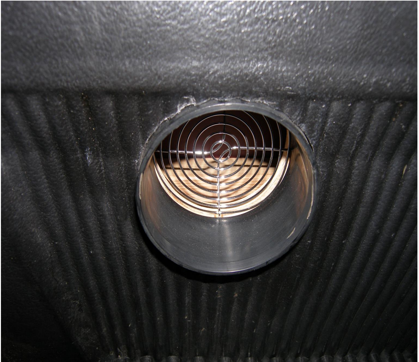
Figure 11 – 10 Detail installation showing grill and shroud but no fan.
