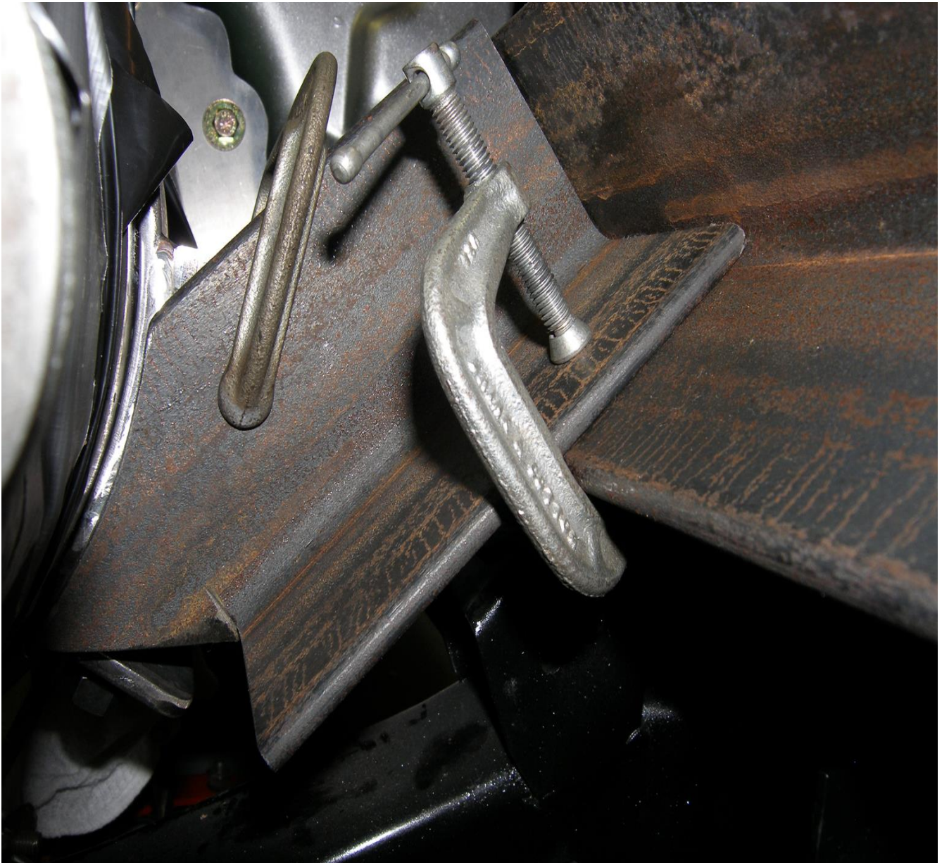
Figure 6 – 5 Detail of the temporary clamps.
