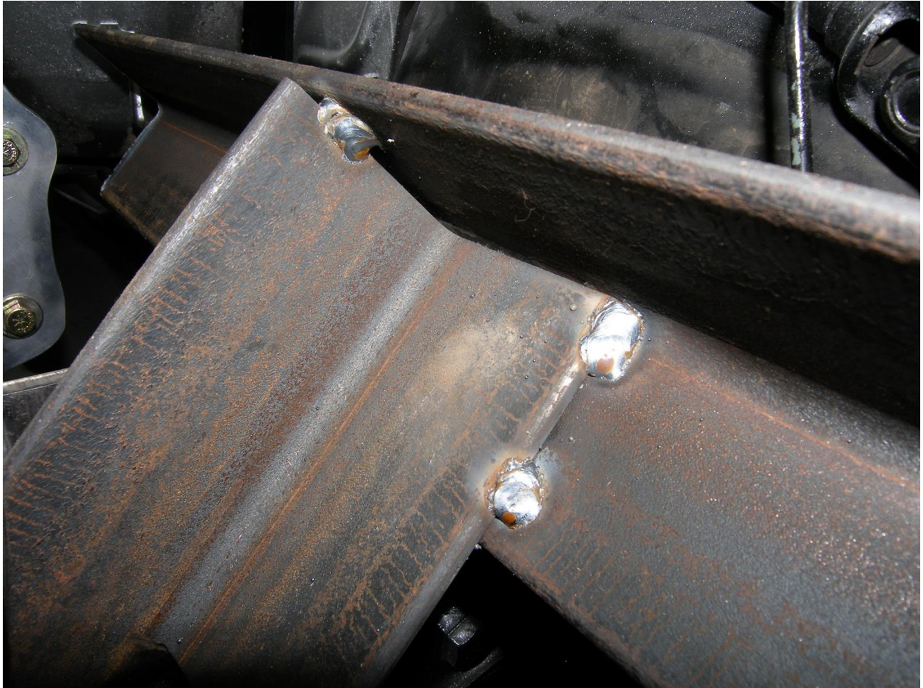
Figure 6 – 8 Detail of spot welding in place.
