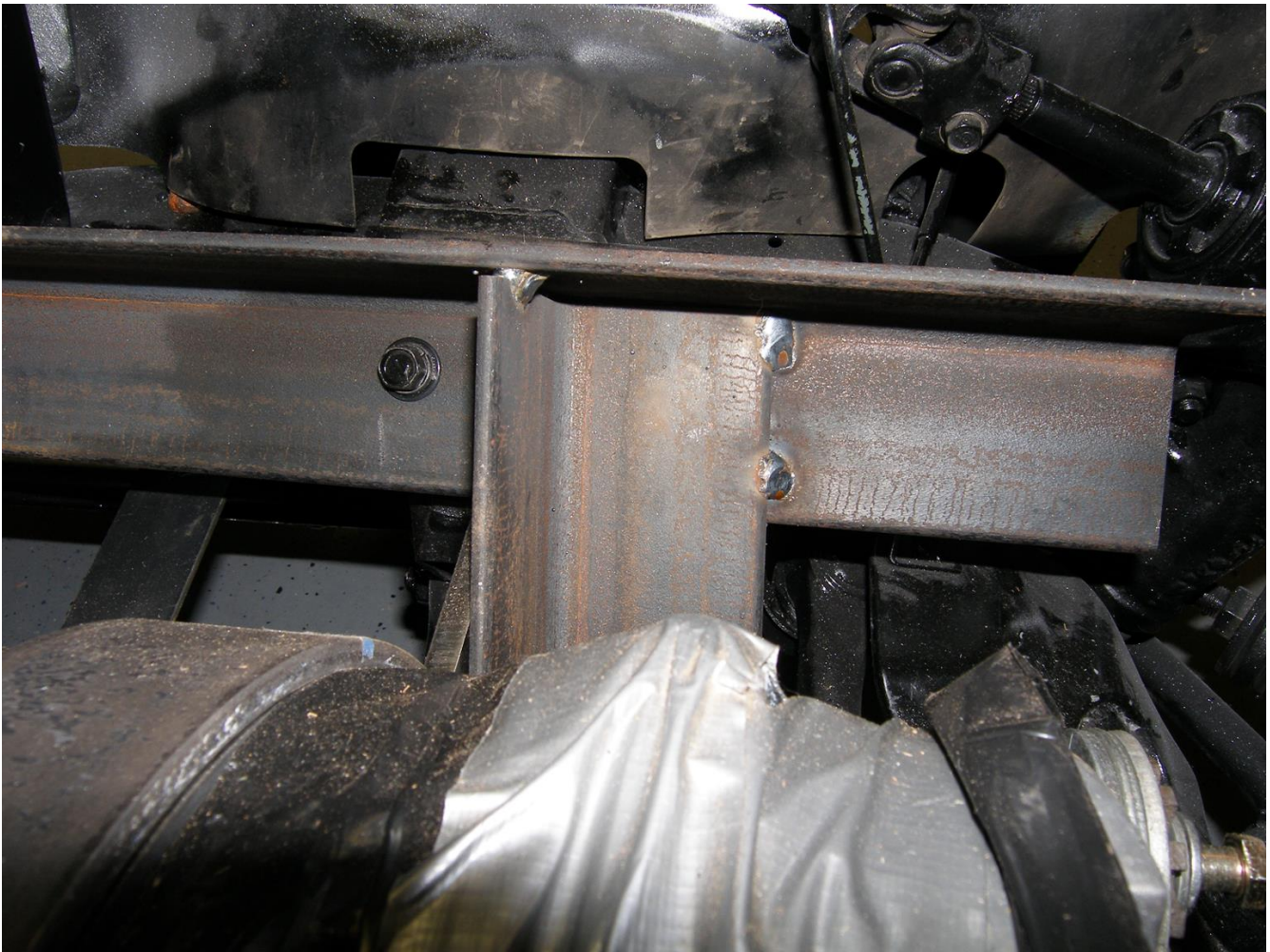
Figure 6 – 9 Spot welds in place plus one bolt shown from base plate to Isuzu motor mount flat.
