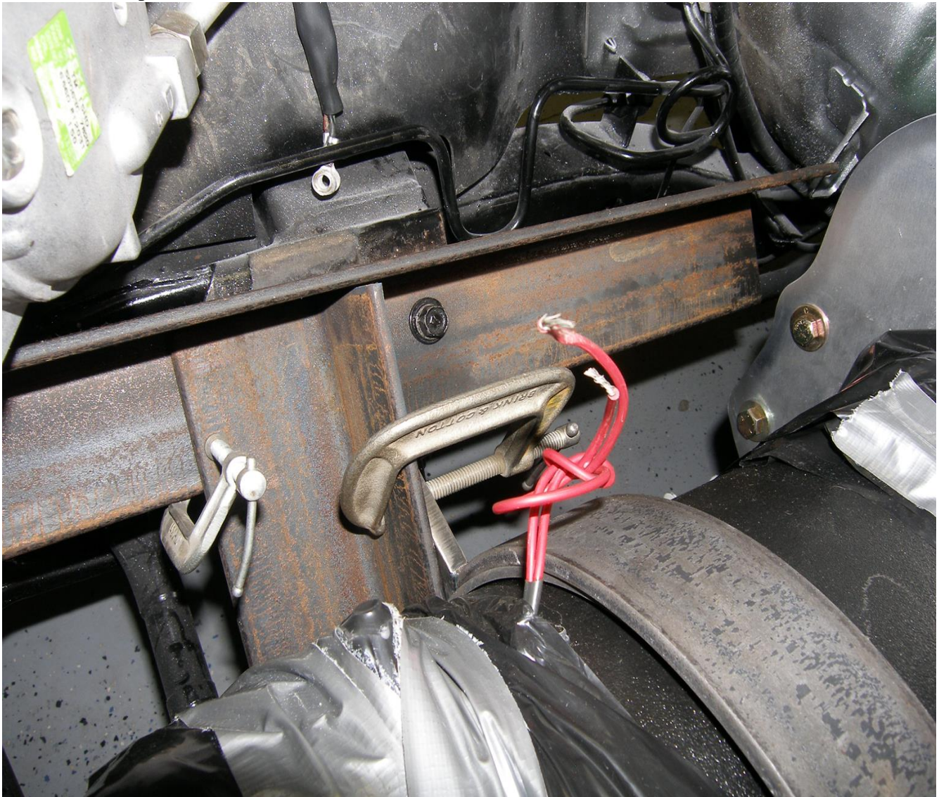
Figure 6 - 4 Temporary assembling of the motor mounts to the motor tabs..
