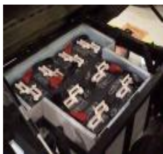
Figure 3 – 7 Inside of truck frame.
